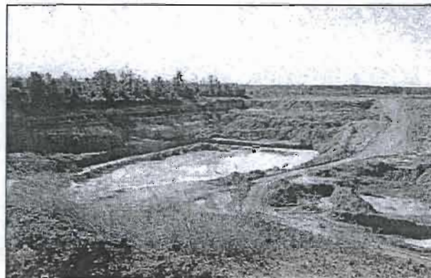
Figure 2. Typical open pit fuller's earth mine near Ochlocknee, Georgia, showing the excavated surface of the minable clay under approximately 20 m of overburden. Ore zone thickness is approximately 4 m.
