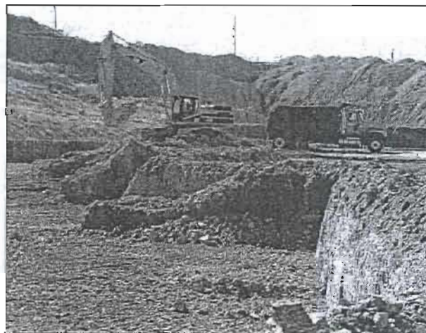
Figure 3. Mining fuller's earth clay after overburden has been removed and hauling by highway truck to the processing plant. Note overburden in the background that has been backfilled to fill the previously mined-out pit.
