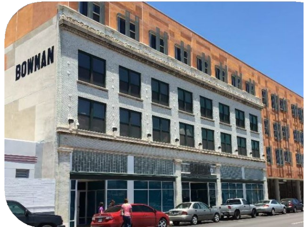
The previously vacant Bowman building was converted to senior housing in 2016 by Nogales Community Development. Image Credit: Manuel Ochoa
