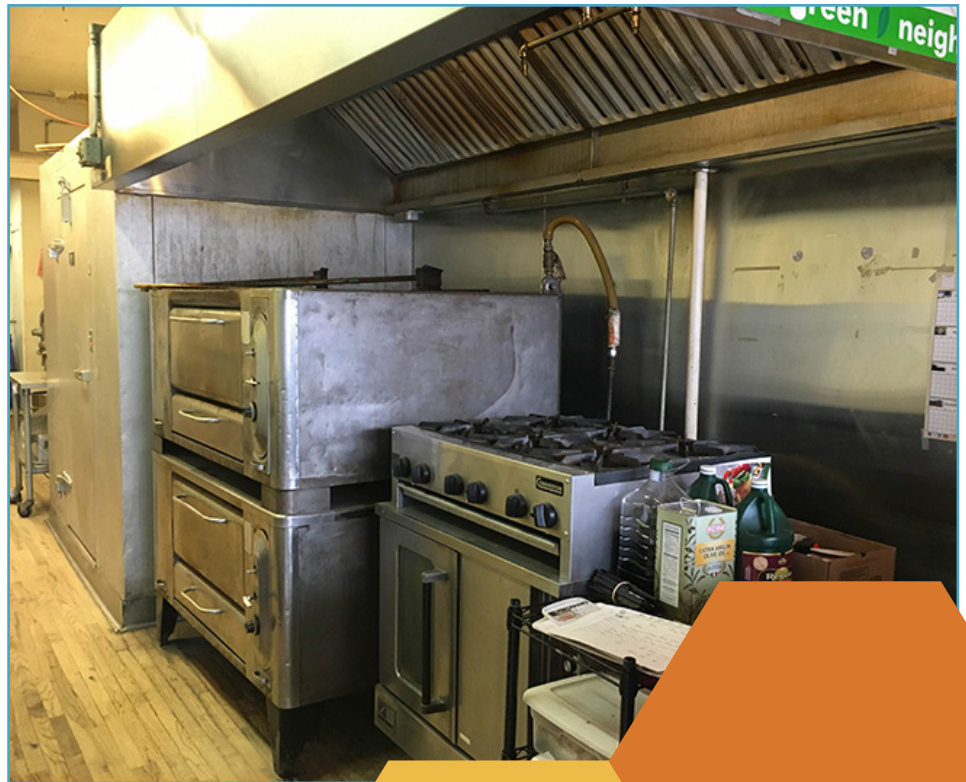
Commercial shared-use kitchen located at Basil Doc's Pizza in Denver, CO, October 2015.
